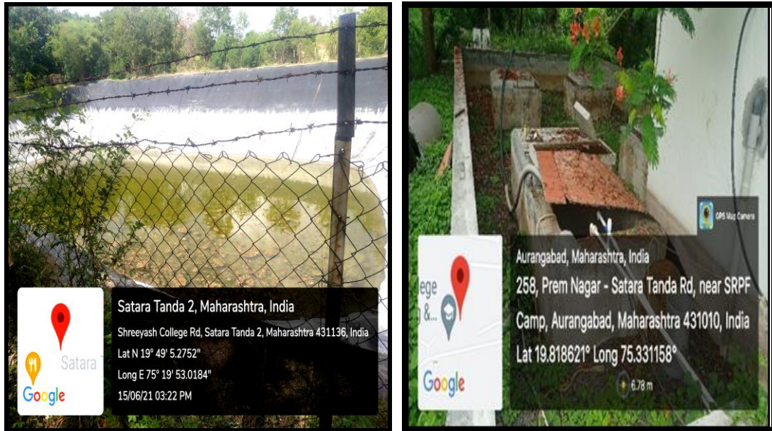
Fig. 7.1.4.4: Sewage Treatment plant (STP) Setup in the Campus
