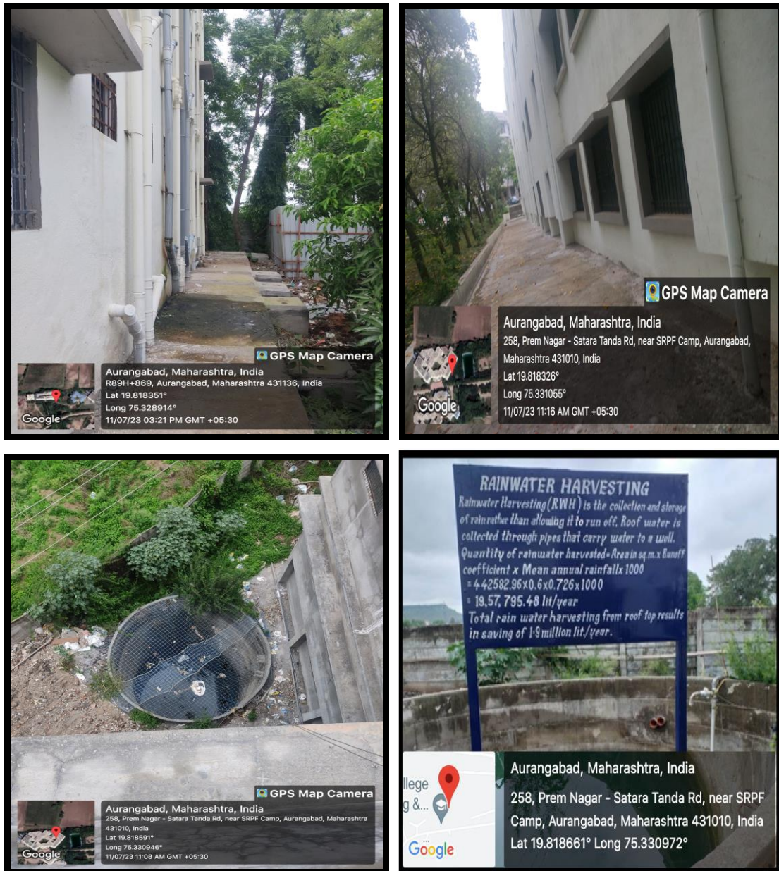
Fig.7.1.4.1: Rain Water Harvesting
