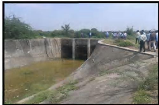
Observing working & component part of Syphon
