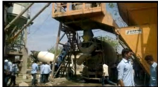
Mixing & filling of RMC in Truck...
