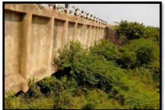
Explaining the component parts of Aqueduct
