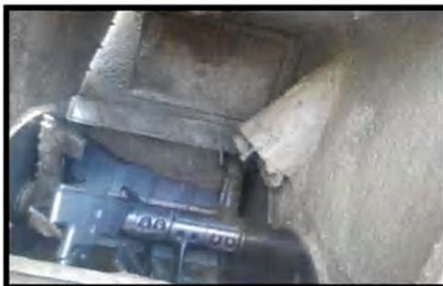
Inside of the RMC plant machine...
